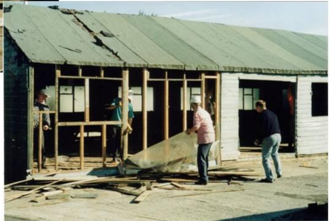
Out Come The Walls
