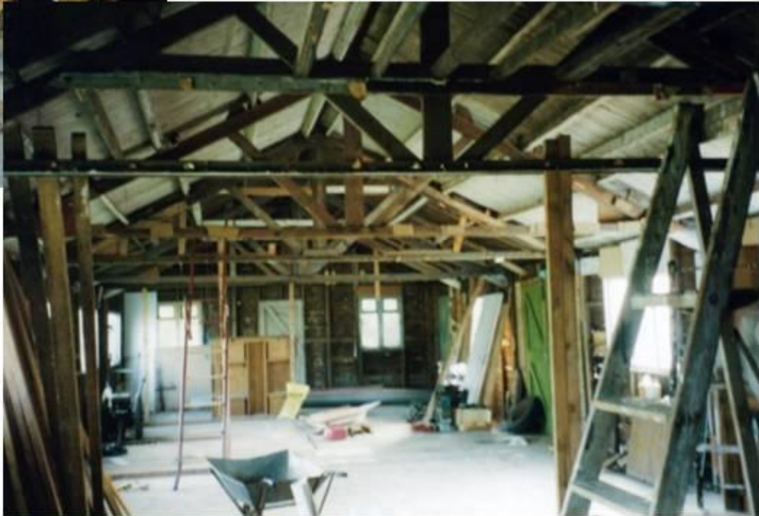
Gutting The Interior
